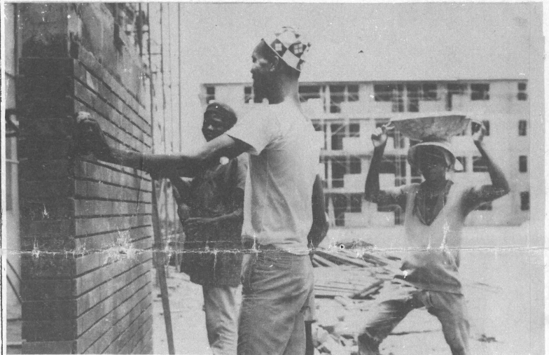
Workers on duty at the construction site at the Festival Village.
